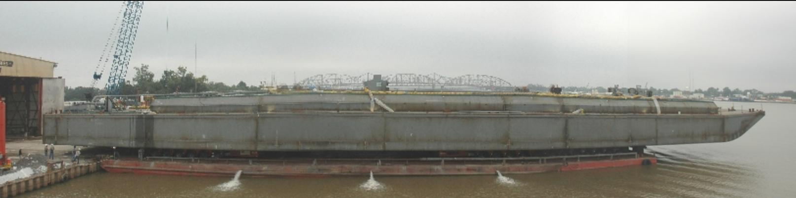
If it were three feet longer, you could play football on it. This 297' long x 54' wide barge weighing in at 950 tons was loaded out using thirty-eight axle lines of SPMT transporters onto the clients barge for launch when blast and paint are complete. Berard also moved the same size barge at the clients Orange Texas facility earlier this month. The Berard Team carried out the job in one day thanks to their hard work and dedication.
